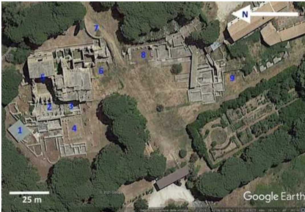
Aerial view of the Taurine Baths. 1. Laconicum, 2. calidarium, 3. frigidarium, 4. Peristylum, 5. imperial calidarium, 6. imperial frigidarium, 7. castellum aquae, 8. Biblioteca, 9. hospitalia and cubicula. Google Earth image 2021.
